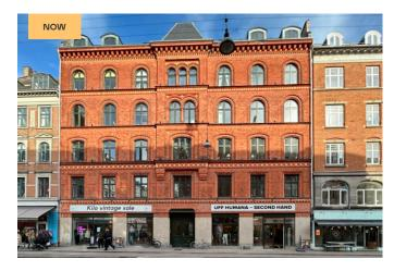
We removed old signs and attached panels from the storefront and renovated one half of it. Unfortunately, we were unable to find any of the original facade under the other half, so we rebuilt it from scratch using handmade stones. Finally, new window sections were installed throughout the storefront. The work was carried out by skilled and proud craftsmen who meticulously cleaned. reused, and rebuilt - all with great respect for the property's character and qualities.
